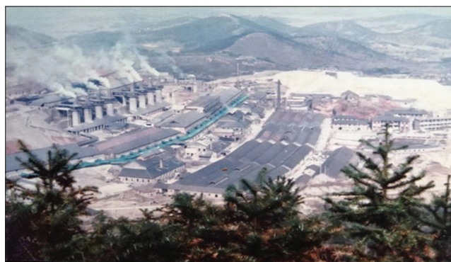
Figure 2. Industrial alum mine production facility Source: Provided by fanshan historical and cultural exhibition hall
